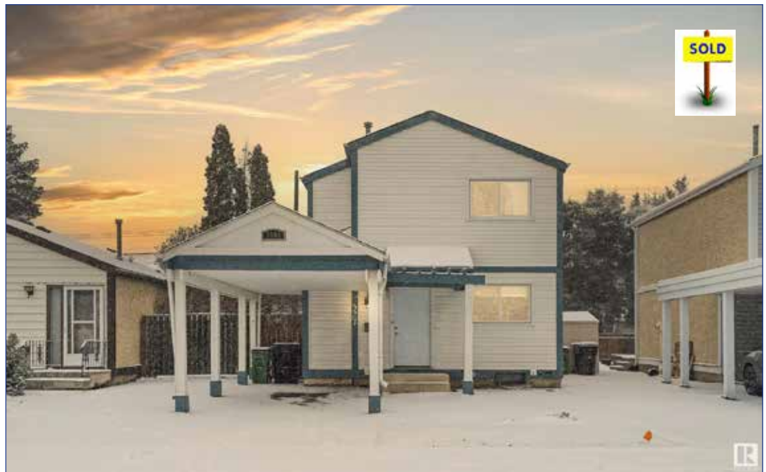
Ottewell: Excellent Starter Home, 3 Bedrooms, 2 Bathrooms, Fully Fenced Yard.
